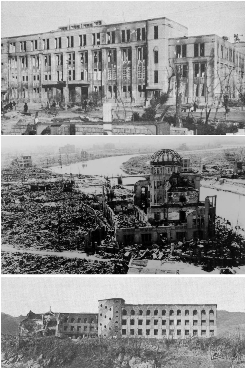
Figure 5.3 Three of many burnt-out buildings that according to various studies [80, 81] yielded pristine tiles or bricks suitable for measurement of \gamma -ray dosage by thermoluminescence. Top: Hiroshima City Hall; center: Hiroshima Prefectural Industrial Promotion Hall (now commonly called the 'Atomic Bomb Dome'); bottom: Shiroyama elementary school in Nagasaki.
