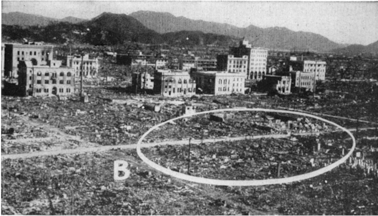
Figure 13.1 Photograph of downtown Hiroshima, taken by Alexander P. de Seversky during his visit in early September 1945. The original figure caption [5] reads as follows: “A cluster of concrete office buildings, standing erect and structurally intact amidst the ashes of the surrounding wooden houses, near ‘ground zero’ (B).”
